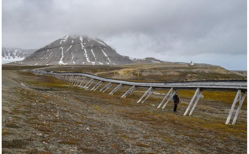
**Figure:** Damaged water pipeline due to thawing permafrost in Norway. CC-BY-NC-ND Rakesh Rao / Climate Visuals Countdown
